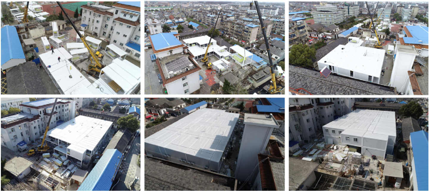
Figure14:Lifting containers in place
