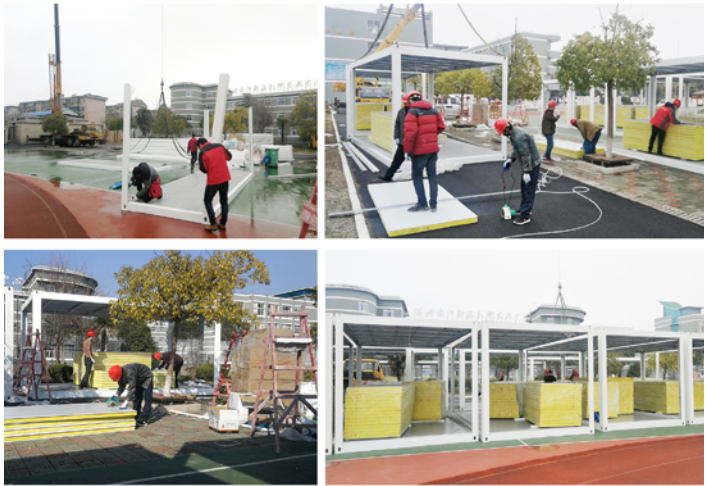
Figure13:Assembling Containers
