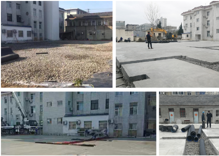
Figure12:Pre-buit-in Pipelines
